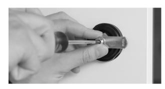
Then check whether the deadbolt gets sufficient hold on the strike plate or the rebate when closed. The latch should be able to be turned to its end position without pressure or resistance when the locking system is closed.
